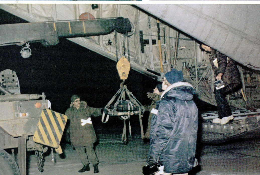
Above. Lead pig used to protect people from 200 R/hr source was so heavy that a recovery vehicle was used to transport it from aircraft to storage area. (EG&G photo 1540-18). Below left. NAST members carefully check the clothing of all recovery team members to ensure it is not contaminated. (EG&G photo 1522-20). Below right. NAST member checks Snowdrift natives for contamination. The results in all cases were negative. (News of the North photo)
