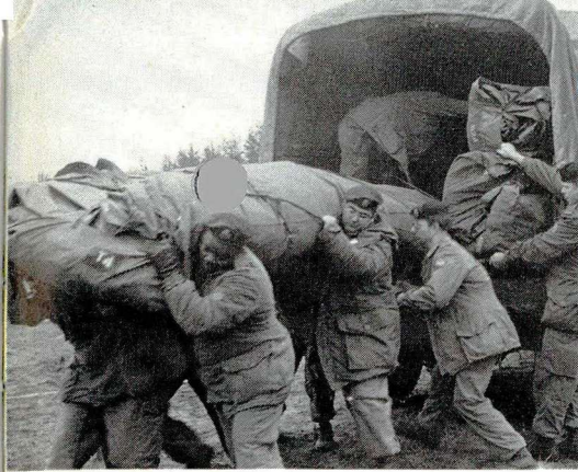
Ease of assembly is the keyword with MUST. An experienced crew can off load and assemble a compartment and connect air, water and electrical lines in less than 30 minutes.
