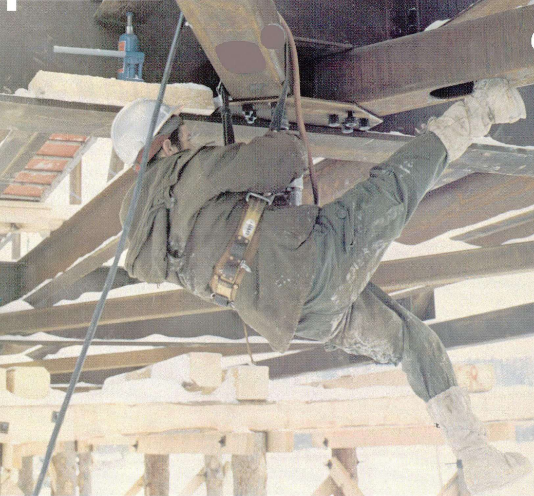
Above. Sapper Mike Gardiner hangs by his safety belt to torque nuts. (REC 77-204) Middle. The bridge site in the summer of 1976 (REC 76-116). Below. Freeze-up has provided the foundation for other false work, on which the first steel is being laid. (REC 77-116)
