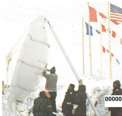
Above. Lt Mike Bolohan of 1 CEU gamely dips his hand for a sample of water from Cosmos Lake. A couple of minutes later he had to break surface ice with a pick to continue the job. (ISC 78-1060). Below. Camp Garland's communications problems were solved by a Telesat Canada earth station. In the camp's early days, communications were restricted by the whims of the ionosphere. With the introduction of the terminal, anyone with a telephone could talk to Camp Garland via Canada's Anik satellite. (ISC 78-1087)
