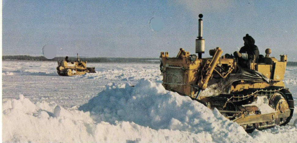
Above. Hardpacked snow, wind-driven to the consistency of concrete, was difficult to move. Heavy equipment operators braved the extreme cold from dawn til after dark for eight days to clear the strip. (ISC 78-1062)
