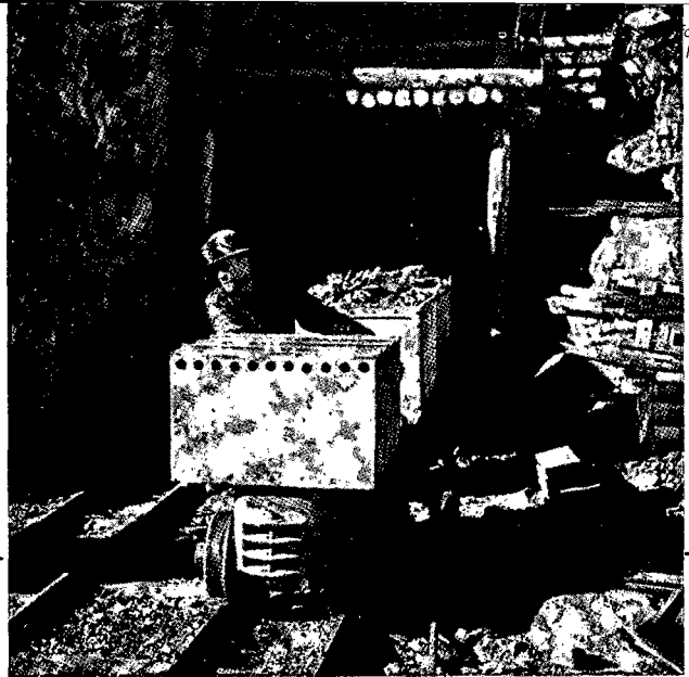
Battery locomotive hauling ore cars from the adit.
