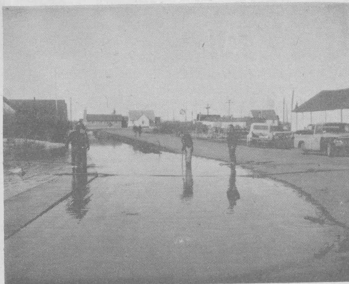
Shown here are workmen thawing culverts with steam to provide drainage. A sudden rise in temperature a short time ago has made it necessary to take such action.
