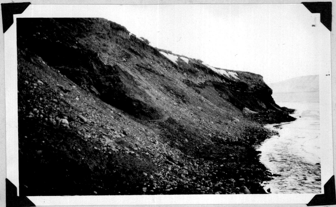
No. 2 - Mine previously driven by Mistaken Chief now in dangerous condition owing to lack of timber support.
